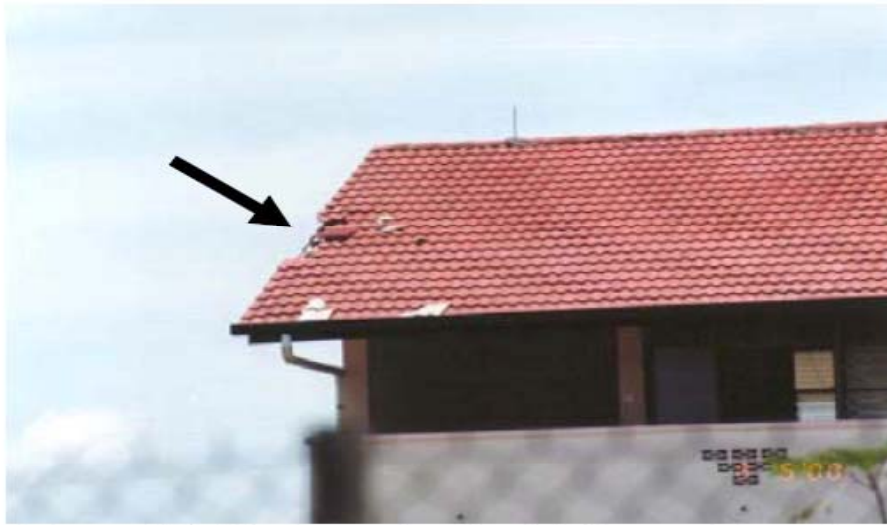
Figure 10: Photograph of a stricken point on the slanting edge of the gable roof. The air terminal conductor should also be installed on the edges of the gable roof.
