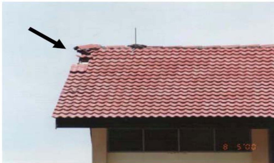
Figure 9: Photograph of a stricken point at the gable roof ridge end. The Franklin rod should have been installed right on top of the ridge end instead of about 1m away from it.
