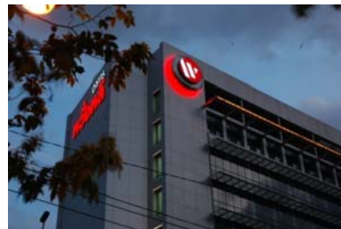
Wang Lee Building
