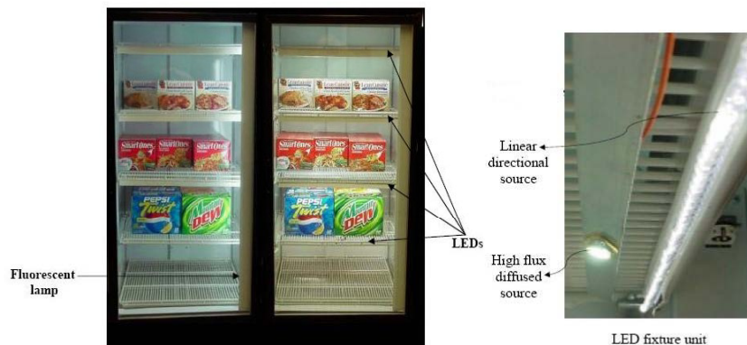
Figure 5: Arrangement of the LED fixture
