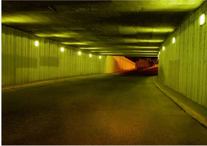
Tunnel Application: Approximately 27.6 m long, 7.6 m wide
