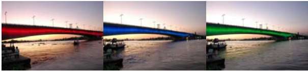
Project : The RAMA IV Bridge
