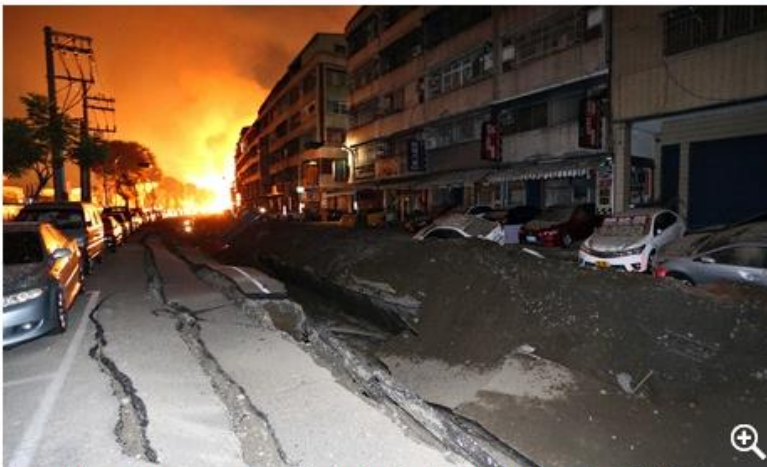
Devastation caused by a gas explosion in Kaohsiung. Photograph: /AFP/Getty Images
